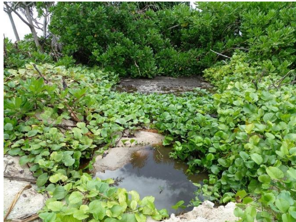
Figure 3: Existing Raw Septage Discharge Point in Shallow Pits at North Lofeaigi
